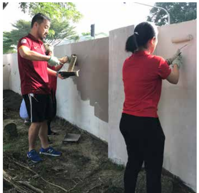
The school compound being brightened by a fresh coat of paint.
